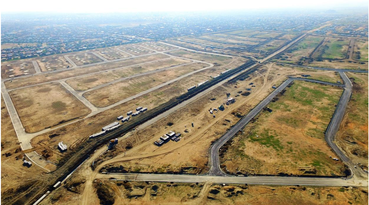
Services installation at Hillside View
